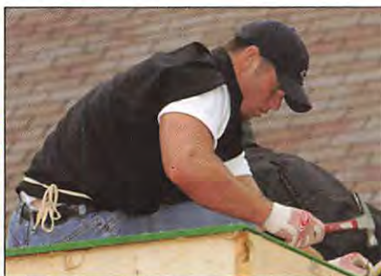
Brant Boyer helps build a home for Habitat for Humanity.
